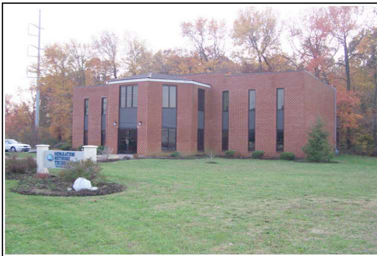
Separation Methods Technologies' 10,000 square foot corporate headquarters in Newark, DE
